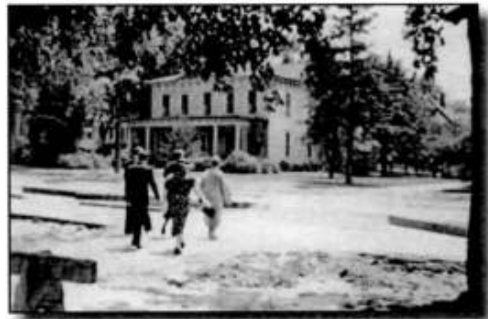
East Main Street under construction in the late 1940's Photo by Delos H. Wray Sr.
