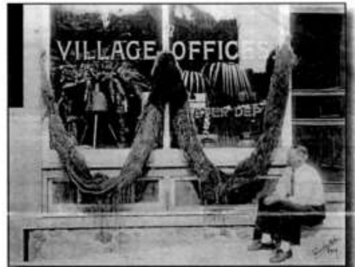
Photo of William Harmon Clark (Supervisor of the Avon Water Works Dept. and father of Relly S. Clark) with big willow root - 24 feet long, taken out of 10" wood water main at Lakeville, 1919. Photo by Pemberton, courtesy AP & HS archives.
