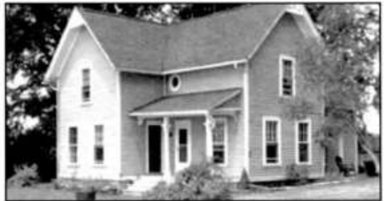
Victorian tenant house, Barber Road, 2017
