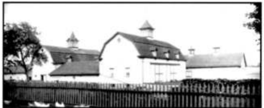
Barn complex, 1920. Source: Mulligan family collection.
