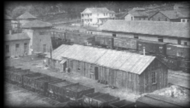
Photo of the Avon rail yard, posted by AP&HS, 18 Mar. 2017.
