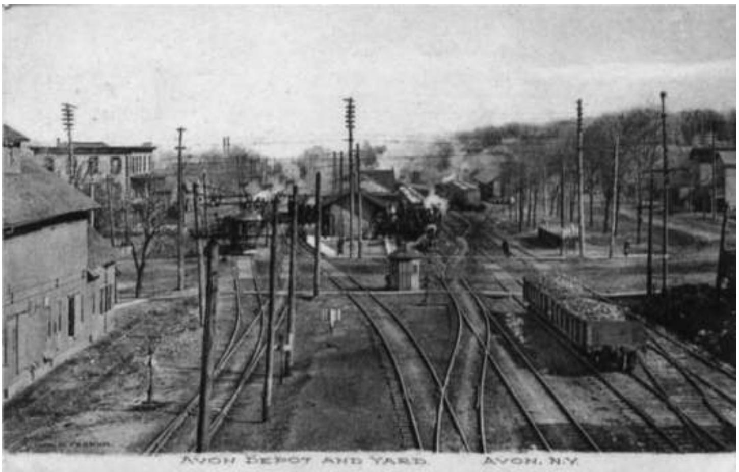
Pattee House and granary on left, freight station in front of passenger station in middle of photo, and Rochester Street on right. Photo was most likely taken from the top of the coaling tower for locomotives. Trolleys to the left of the station date this photo to c. 1907.
