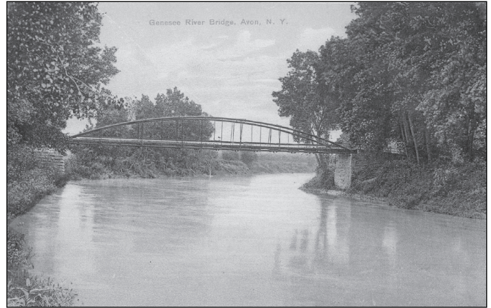
Genesee River Bridge, Avon, NY
