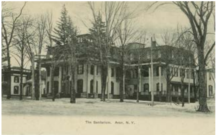
In 1882 the building was expanded to host its first business, adding a west wing, third floor and a cupola. Source: Avon Town Historian
